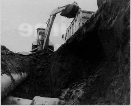
Many times, backhoes are used not only for excavating, but also for loading the displaced dirt into trucks for transport elsewhere.
