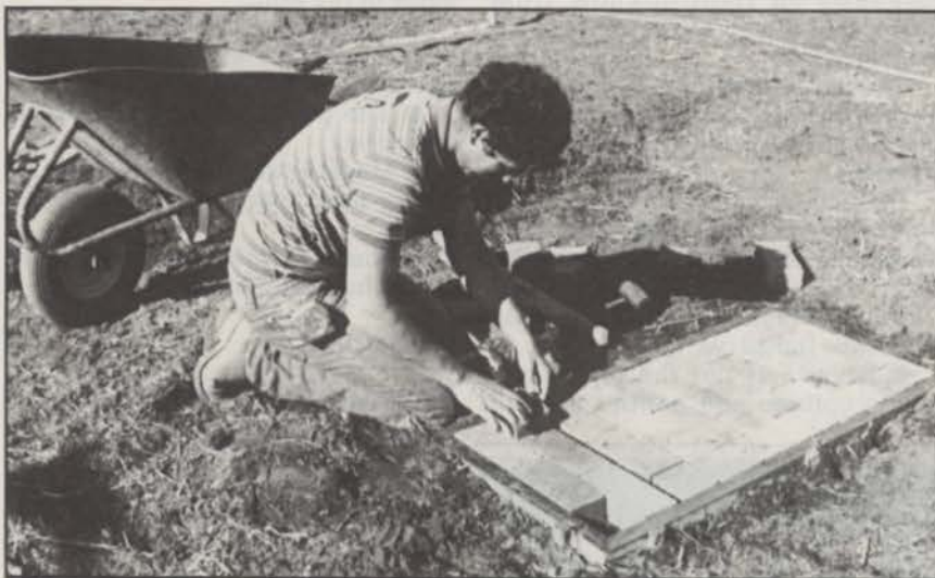
A candidate sets bricks in a running bond pattern according to specifications in the brick-on-sand portion of the CLCA's certification test. The exam took place last October at Football College, Los Altos.
