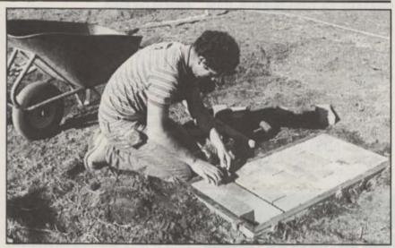
A candidate sets bricks in a running bond pattern according to specifications in the brick-on-sand portion of the CLCA's certification test. The exam took place last October at Football College, Los Altos.
