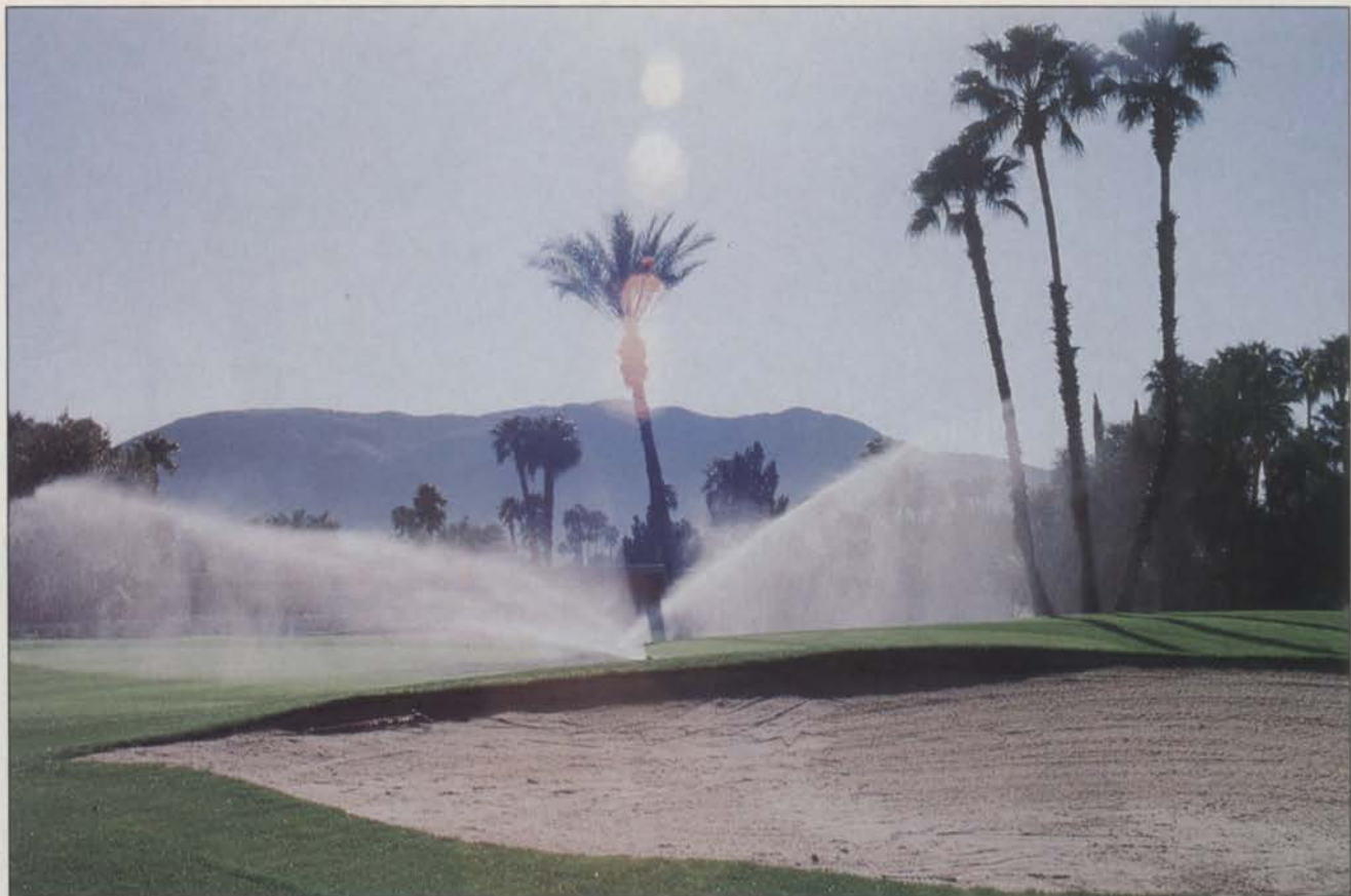
This water-efficient low-pressure irrigation system at Canyon Country Club is also a money-saver.
