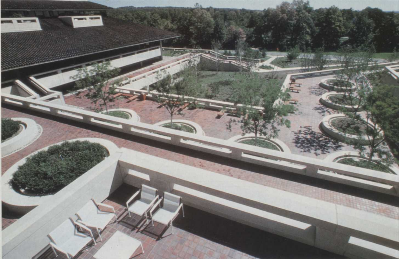
A view of the courtyards at AT&T's Basking Ridge site. There are 1,200 trees on the 126 acres of land.
