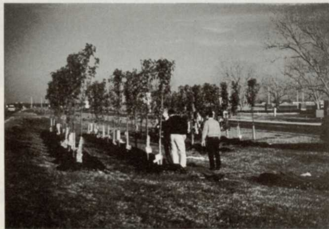
A portion of Highway 90-A's median
