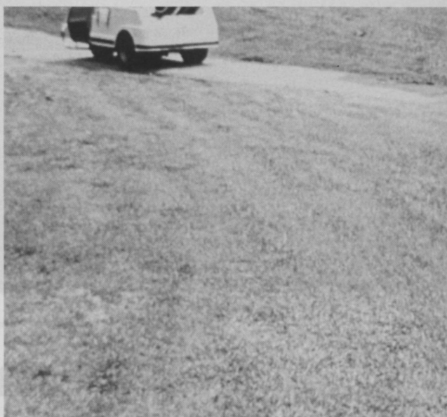
Biltmore Forest Country Club superintendent Don Burns notes the problem he had with the cart path on the number 8 hole (left). At right is the much-improved path after using Enkamat.
