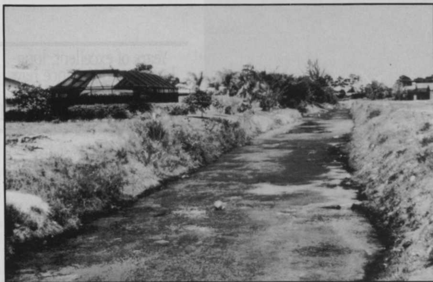
Aquatic weeds may reduce or severely restrict water flow (as much as 90 percent) in irrigation canals and drainage ditches.
