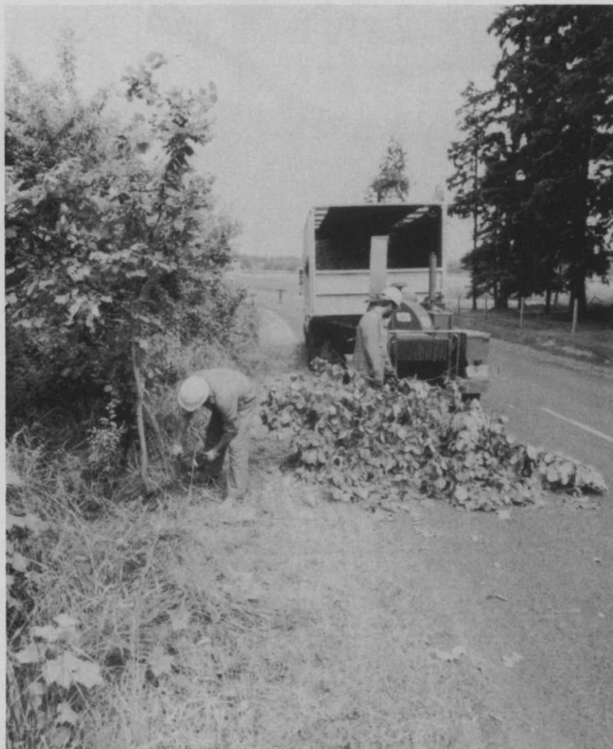
Workmen clear brush from right-of-way area.
