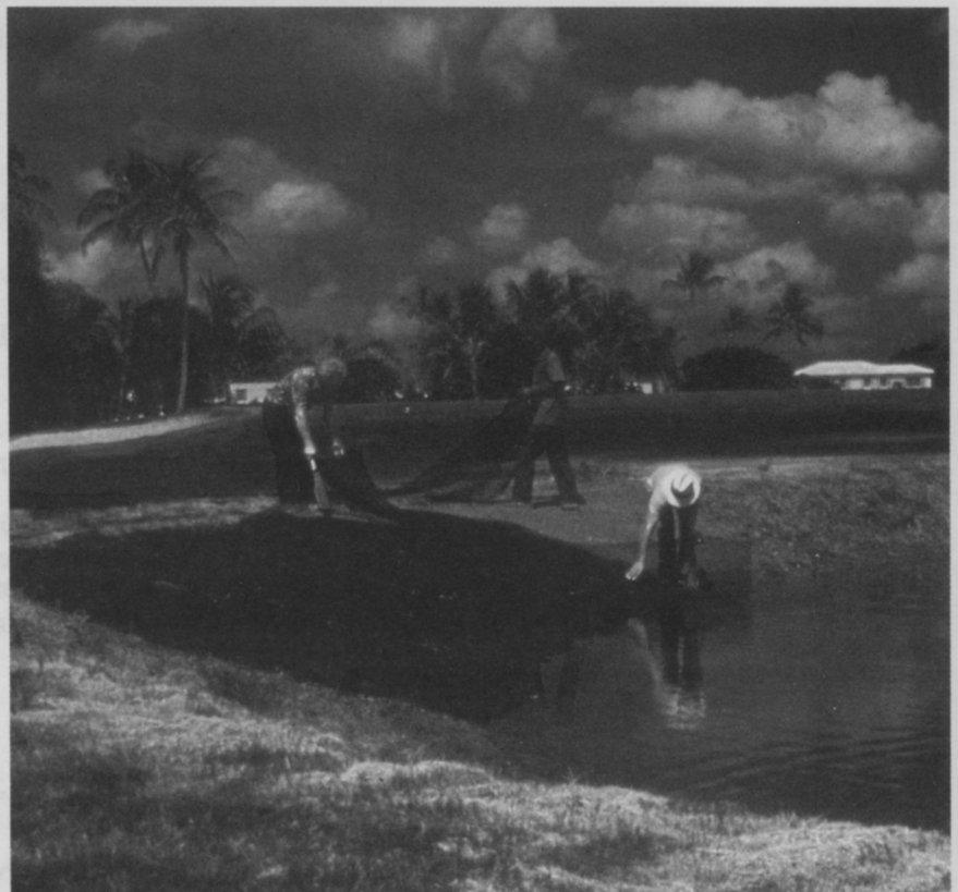
Workers install Enkamat to prevent erosion of a pond's bank.
