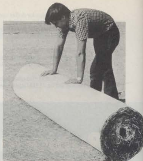
While installing North American Green's erosion control blanket, one should start at the top of the slope and unroll the blanket. The blanket should never be stretched so that contact with the soil is constant.
