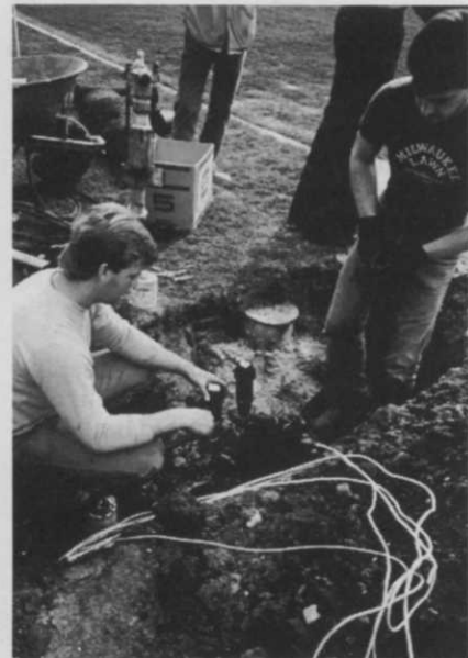
Workers from Milwaukee Lawn install the Toro sprinkler heads.
