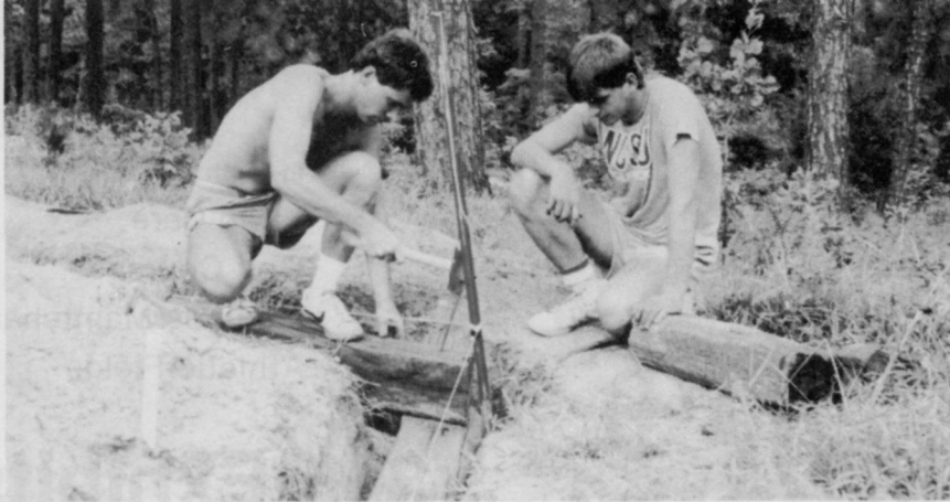
Students Blain Ritter and Jeff Etheridge work on the back retaining wall for the Sir Walter Raleigh Garden.
