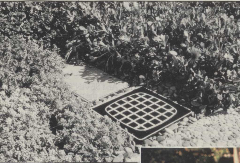
Well lighting is less conspicuous while at the same time providing utility and compactness.
