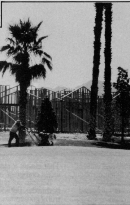
At the Lakes Country Club, Palm Desert, CA, course renovation and construction of exclusive private villas go on simultaneously.
