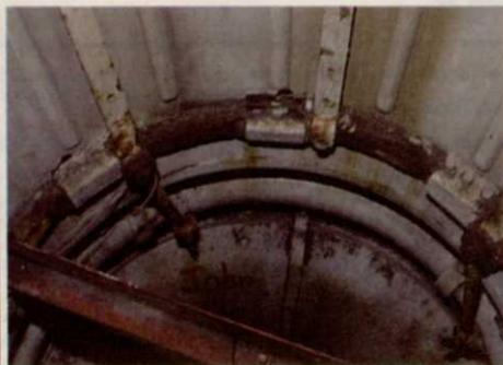
A century of fatigue and corrosion has weakened the Statue's frame, eaten holes in the copper skin.
