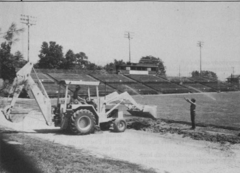
Filling in around irrigation lines at Galbreath Field, King's Island.
