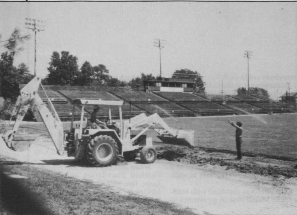
Filling in around irrigation lines at Galbreath Field, King's Island.
