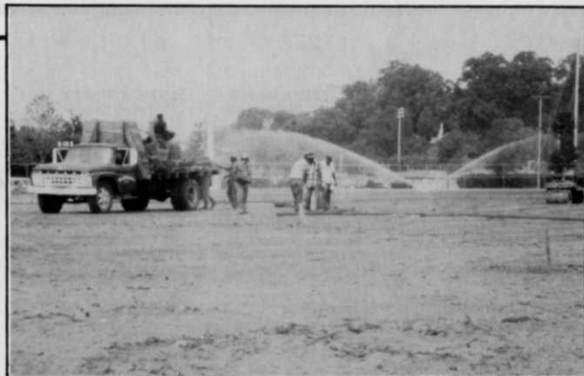
Outside Contractors install new sod after raising the crown of one of the academy's intramural fields.
