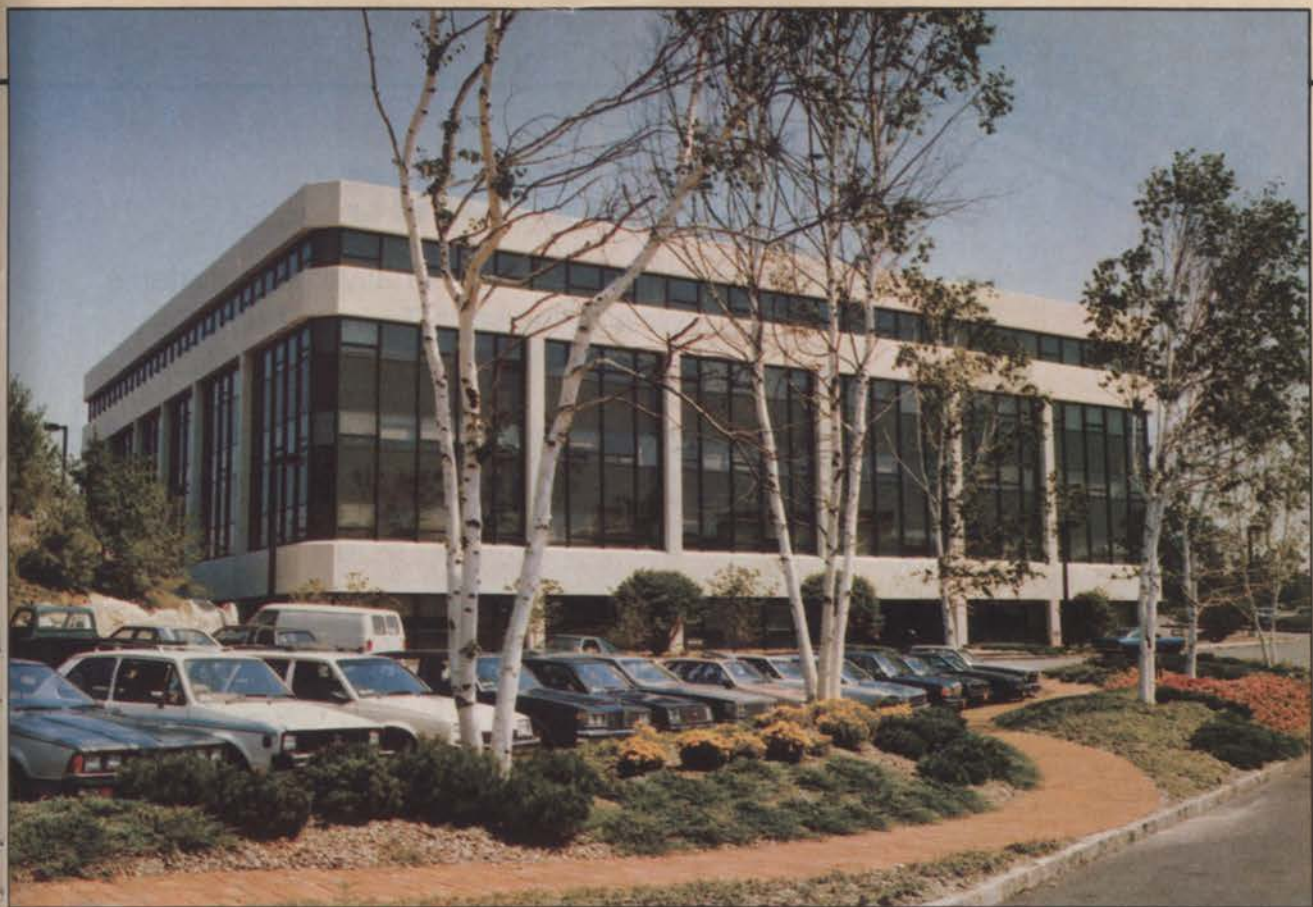
244 Westchester Avenue is a focal point along the Platinum Mile.
