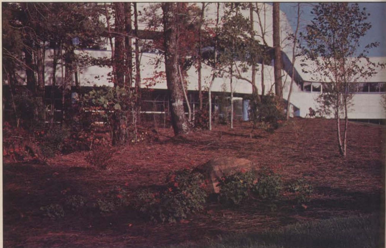
The Union Carbide building sits nestled in a natural setting in Research Triangle Park, NC.
