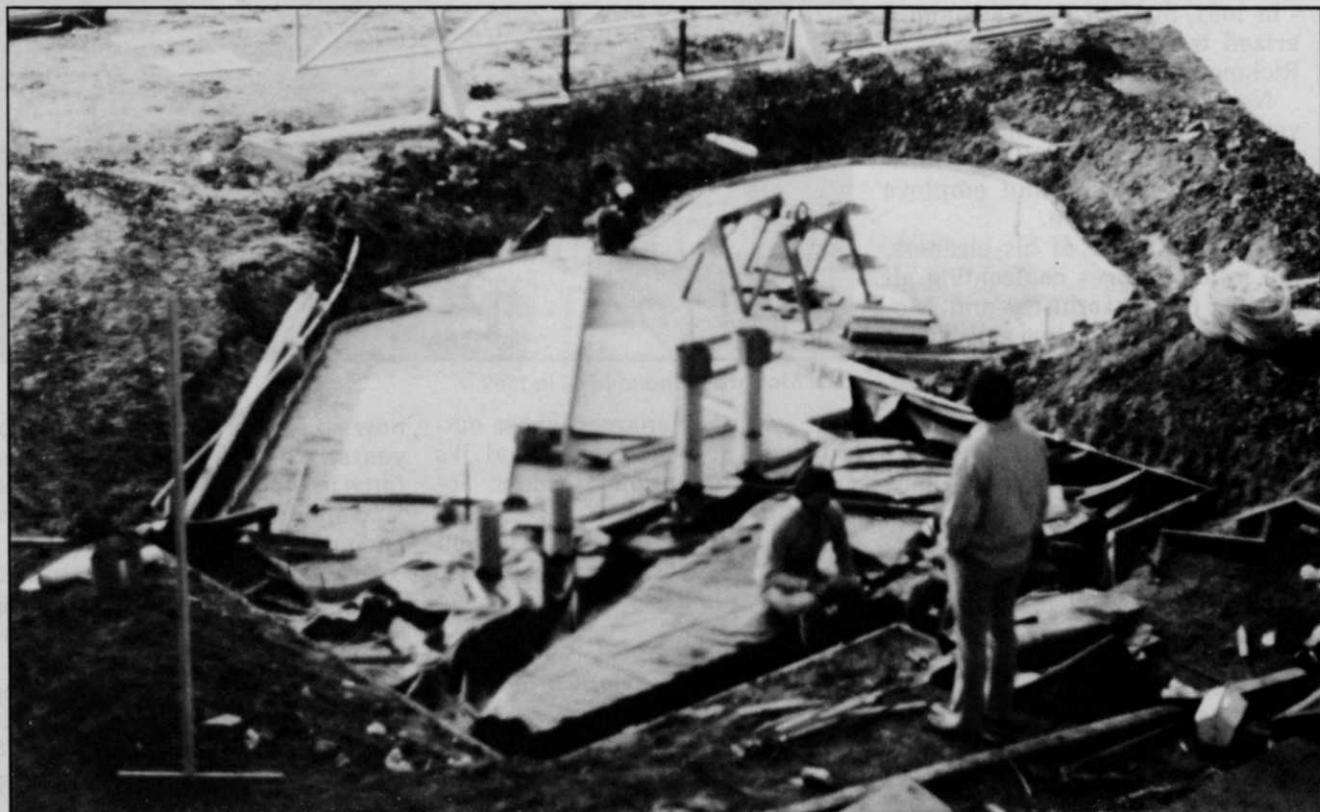
LDC is doing everything but electrical and plumbing at Universal Resources
