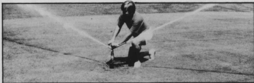
Pakkala locks in head to manual irrigation system. An automatic system is part of the reconstruction plan.
