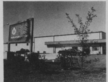
New RIS facility.
