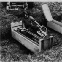
Mole is designed to install pipe up to 8-in. in diameter under streets, roadbeds and other obstructions that cannot
