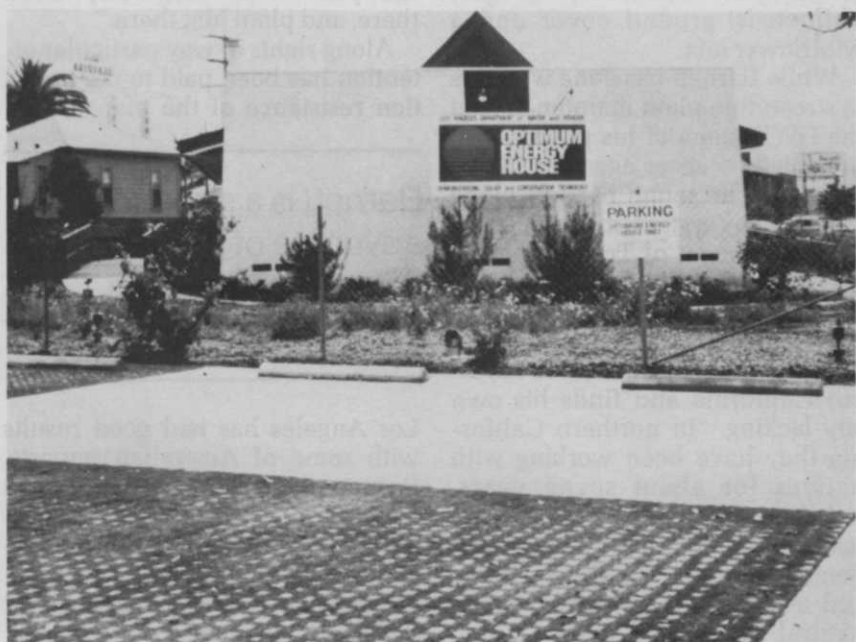
LA's Optimum Energy House not only has a native vegetation landscape, but the parking lot is partially turf blocks to reduce the impact of pavement.
