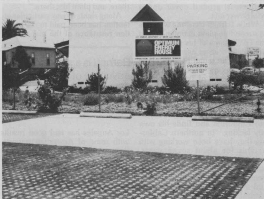
LA's Optimum Energy House not only has a native vegetation landscape, but the parking lot is partially turf blocks to reduce the impact of pavement.
