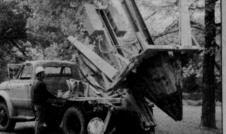
**TS-50M.** Truck-mounted. Outstanding maneuverability. Extension and side-shift features let you hydraulically position the spade an additional 21'' away from the frame and  $151/_2''$  left or right of center.
