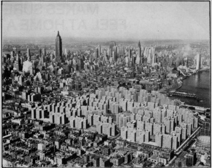
Overhead view of Peter Cooper Village and Stuyvesant Town.
