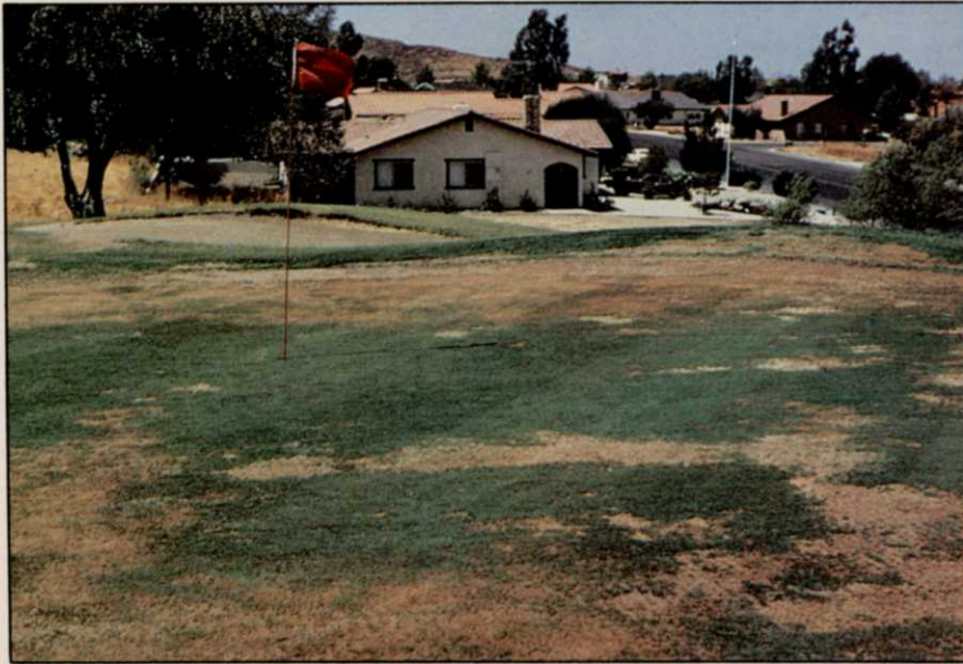
No amount of maintenance can correct severe compaction problems. Redesign and rebuilding may be necessary.
