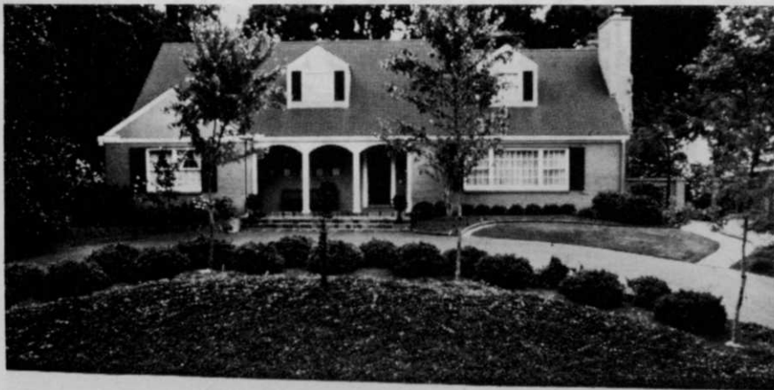
Circular driveway and berm made this simple, boxy house stand out.
