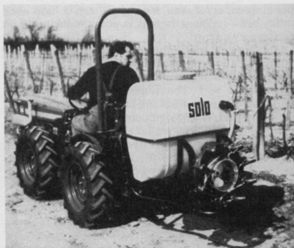
Solo's 451 and 452 Mistblowers apply high-concentrate, low-volume spray and are designed for tractors with horsepower over 18.
