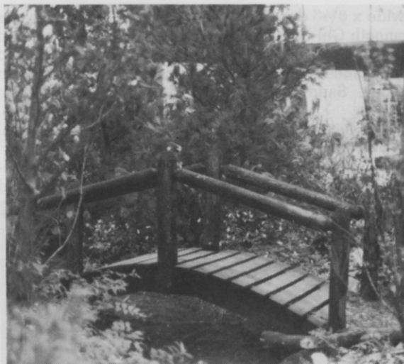
A rustic cedar wood bridge by Valley View of northern white cedar has rot-resistant handrails.
