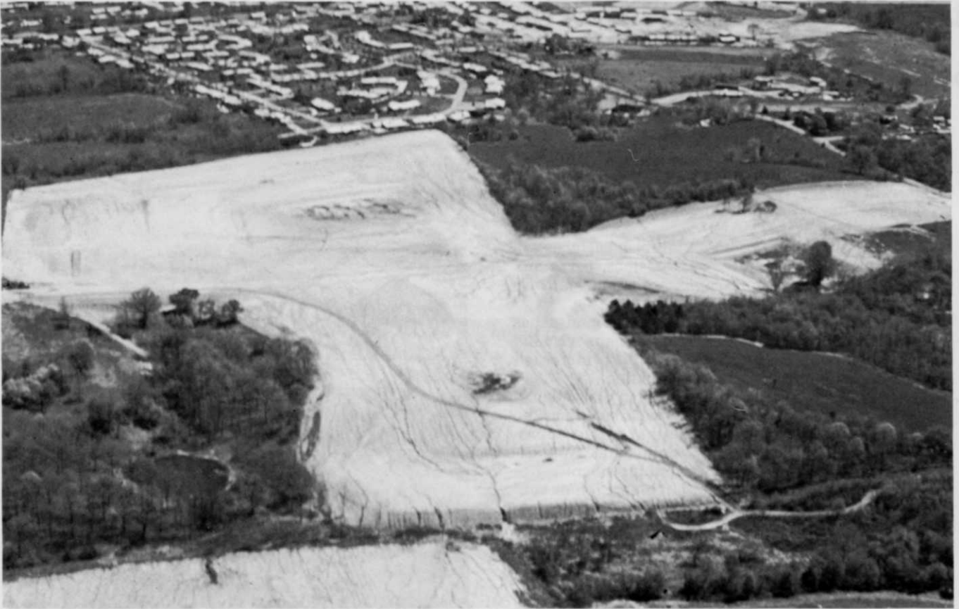
Aerial view of site developed for building shows erosion beginning on smooth slopes. Note rills forming.
