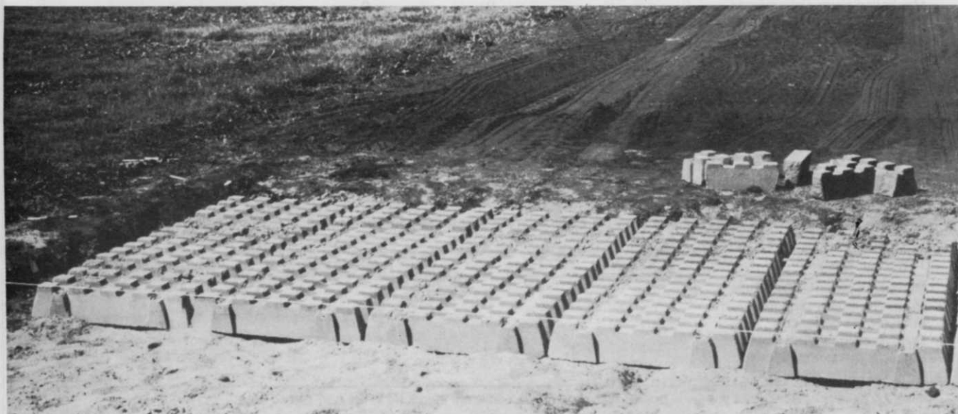
Turf pavers ready for topsoil and seeding in cart path.
