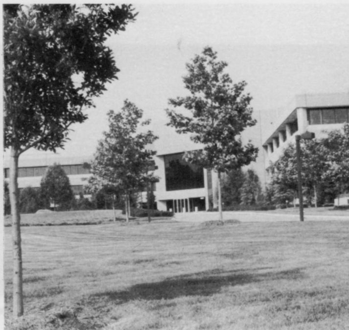
View from entrance of Martin-Marietta headquarters.
