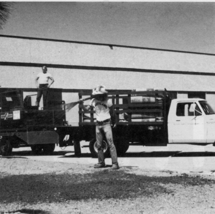
Bowie pull-behind unit in hose operation. The unit requires one person to control the clutch and another to operate the hose.
