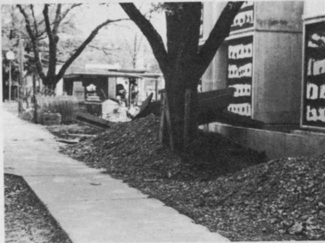
Trunk protection cannot offset the root damage caused by sidewalk and foundation construction. Dieback is already evident before construction is completed.
