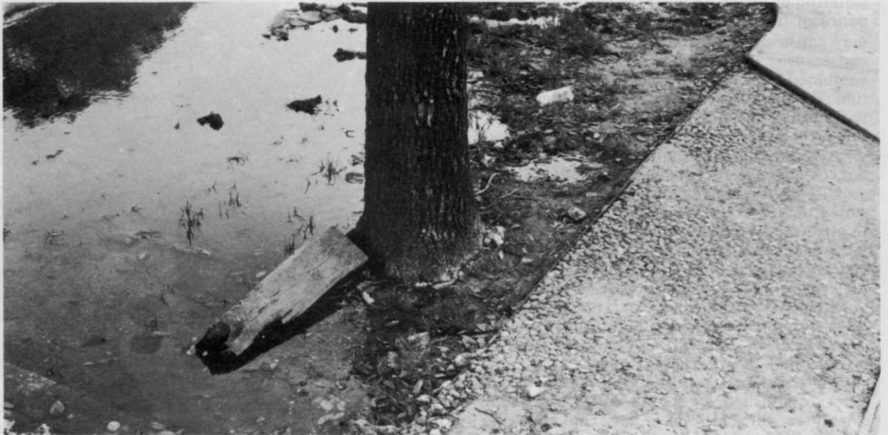
Poor drainage around construction areas can be very damaging to trees.
