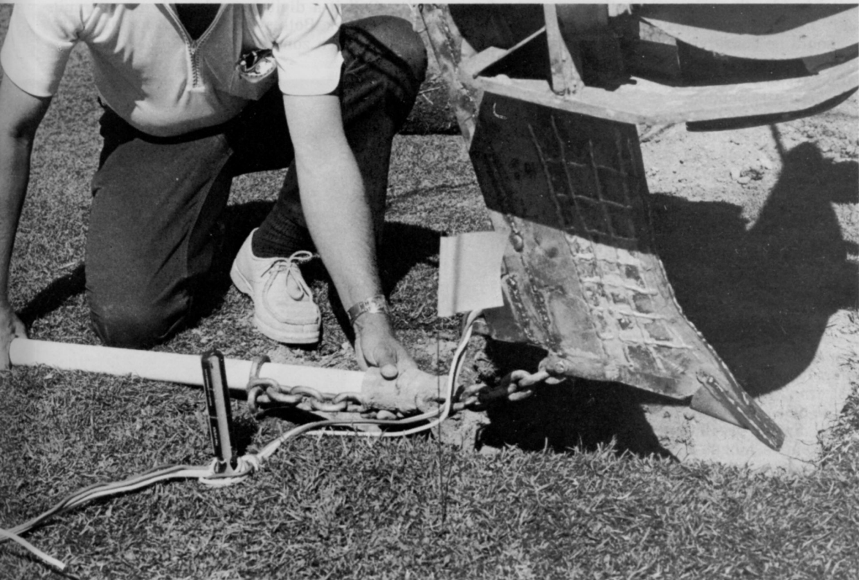
Pulling pipe and wires into ground causes minimal surface disturbance (above). Pipe is attached to vibratory plow blade with pulling grip (below).
