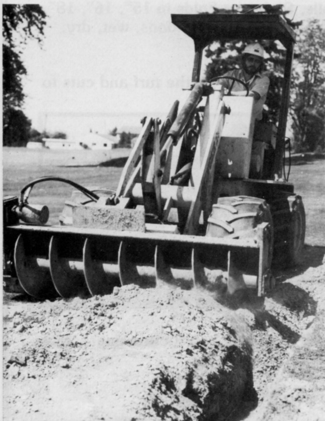
Auger replaces soil where vibratory plow began pipe and wire pulling.
