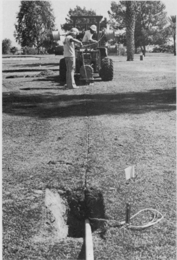
Pulling pipe and wires into ground causes minimal surface disturbance (above). Pipe is attached to vibratory plow blade with pulling grip (below).
