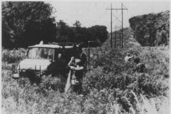
Modern Asplundh crews have more manpower, larger trucks with larger tanks and twin-nozzle hoses for speedier application.
