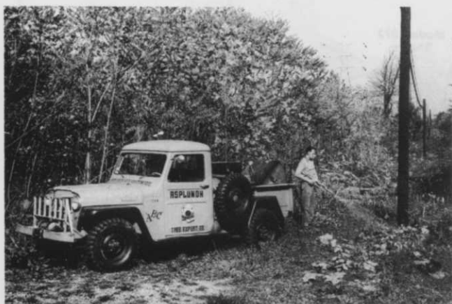
In the early days of electric line maintenance, Asplundh had one-man crews with little equipment
