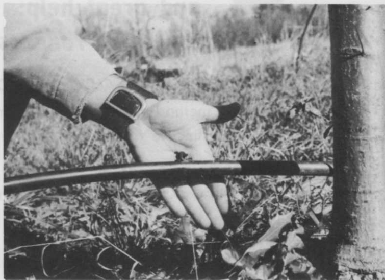
Emitter , inserted directly into laterals through a hole punched at the base of each tree, simplifies and shortens the installation process.
