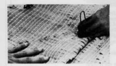
until vegetation is firmly established. Made by Gulf States Paper Corp., Hold/Gro is available in a variety of grades and sizes. The lightweight material can be installed by just two men.
