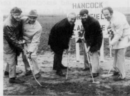
New turf field lab at Michigan State University is now under construction after this ground breaking ceremony in October. The new Hancock Turf Field Lab will centralize all turf research plots at MSU while providing office space. Taking part in the ground breaking are (left to right): Dr. Paul Rieke, Dr. Ken Payne, Dr. Dale Harpstead, Dr. John Kaufmann, and Dr. Joe Vargas.
