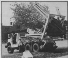
Vermeer Tree Spades. Patented tree-moving/tree-packaging machines that automatically dig, ball, transport and replant shrubs and trees up to 25 ft. in height. Tractor-mounted, trailer-mounted, or truck-mounted units—plus complete multi-purpose landscaping machines that handle a tremendous assortment of dirthandling functions in addition to transplanting trees.
