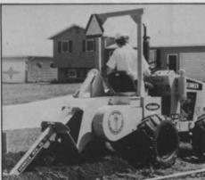
Vermeer Trenchers. Multi-purpose underground machines with a wide variety of money-saving dirt-handling attachments. On tracks or rubber tires. With power ranges from 18 to 195 hp. With digging capacities of 4-36 in. wide, down to 12 ft. deep. Vermeer Vibratory Plows, for installing cable directly underground without damaging finished surfaces or landscapes.
