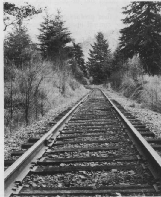
DOT insists that railroads have good visibility and safe operating conditions.
