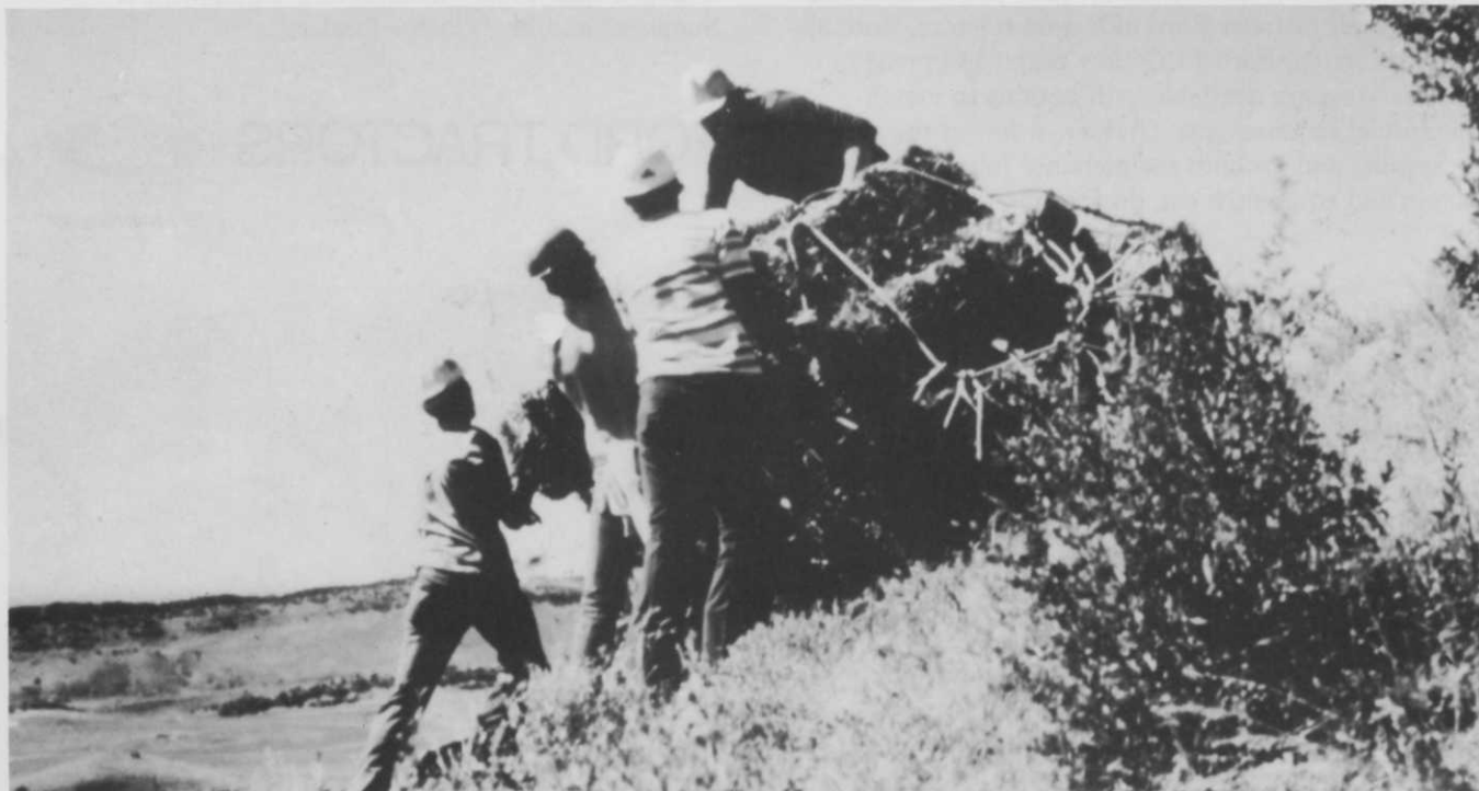
Workmen on hillside unload materials brought to the site by helicopter. Use of the helicopter preserved the slope from additional wear.
