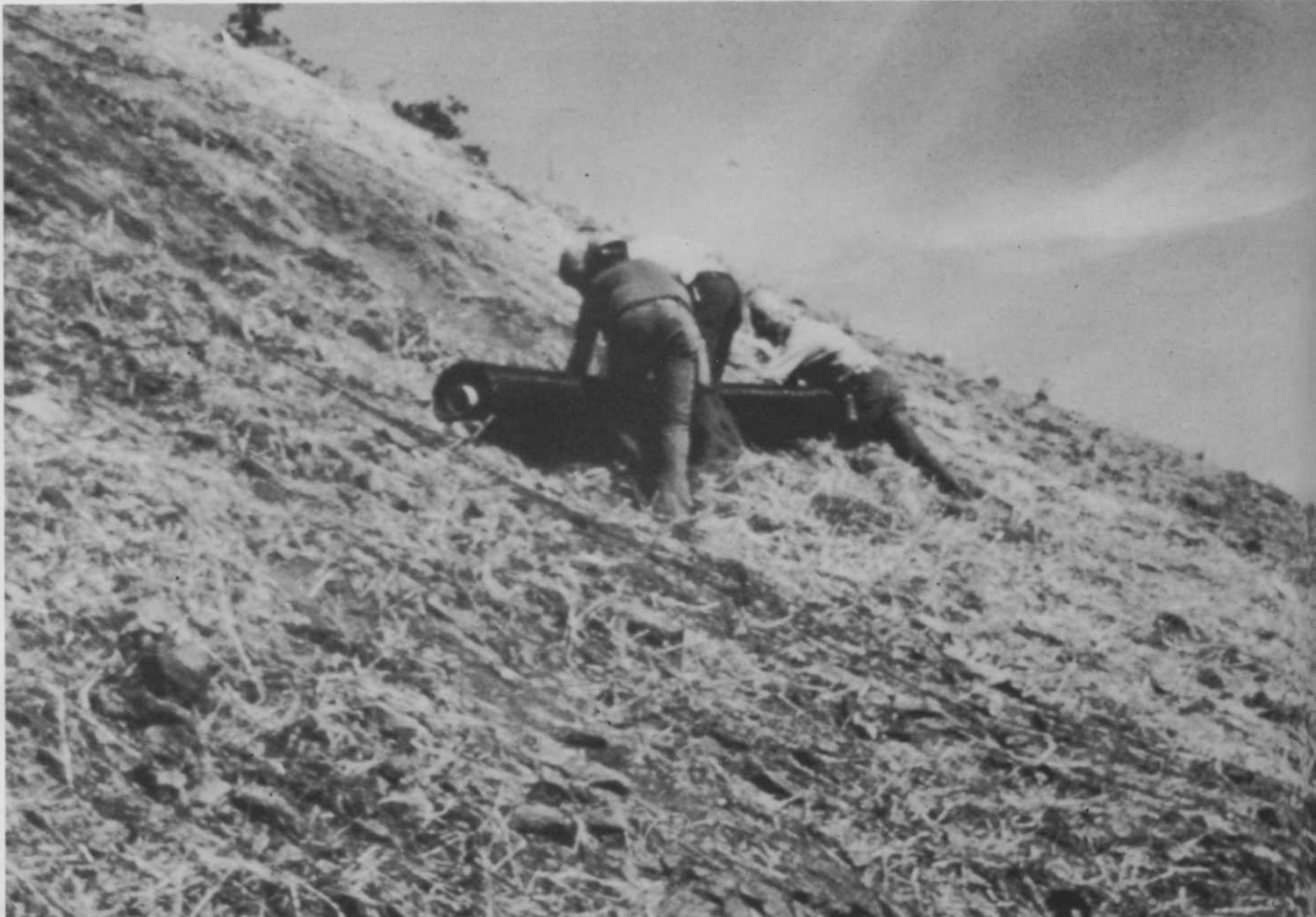
Workmen roll out netting by hand so as not to disturb the relatively loose soil structure of the canyon wall.
