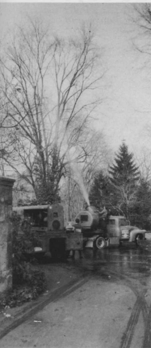
A roto-mist sprayer comes in handy, when more than one side of the tree can be reached with it.
