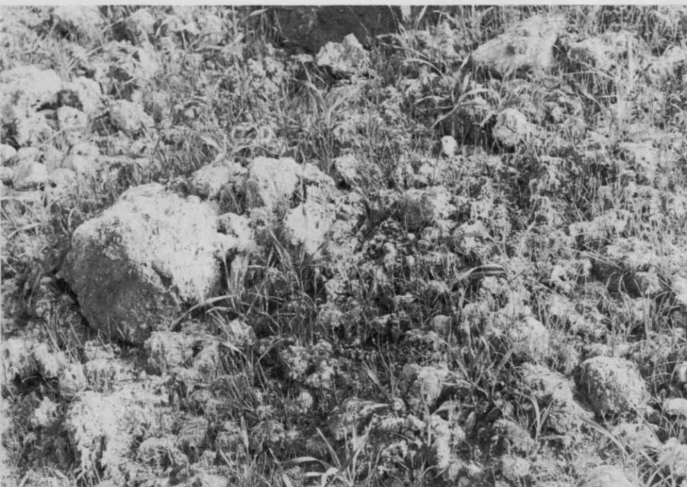
Excellent germination and seedling growth (above) on a 1:1½ fill slope with a rough, loose surface mulched with 1,500 lbs./acre of woodfiber. A roughened 1:1½ fill slope (right) after applying 3,000 lbs./acre of straw and overseeded with a slurry of seed, fertilizer, and woodfiber at 700 lbs./acre.
