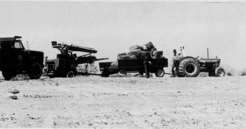
Workers for the Ohio Mining and Reclamation Association prepare to mulch newly seeded area nearby (top). A silt basin (below) is a vital part of mine reclamation and is usually the first step of the reclamation process. Reclaimed soils can absorb limited quantities of rainfall. Therefore, increased runoff must be handled through special ditches and silt basins.
