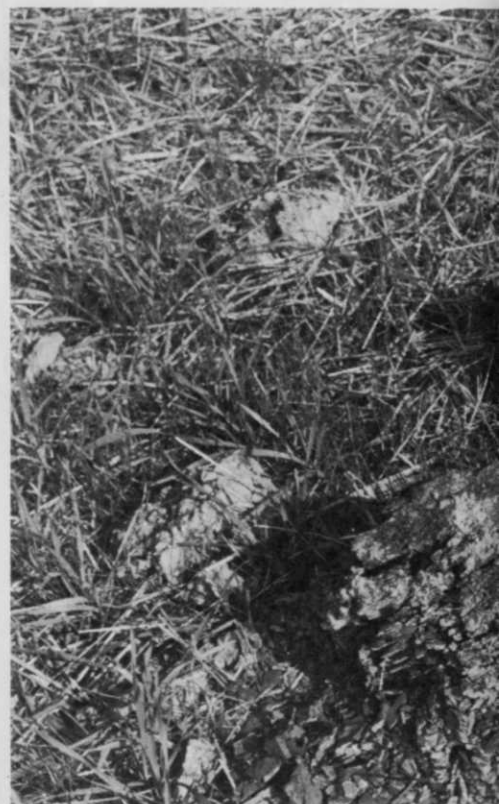
Excellent germination and seedling growth (above) on a 1:1½ fill slope with a rough, loose surface mulched with 1,500 lbs./acre of woodfiber. A roughened 1:1½ fill slope (right) after applying 3,000 lbs./acre of straw and overseeded with a slurry of seed, fertilizer, and woodfiber at 700 lbs./acre.
