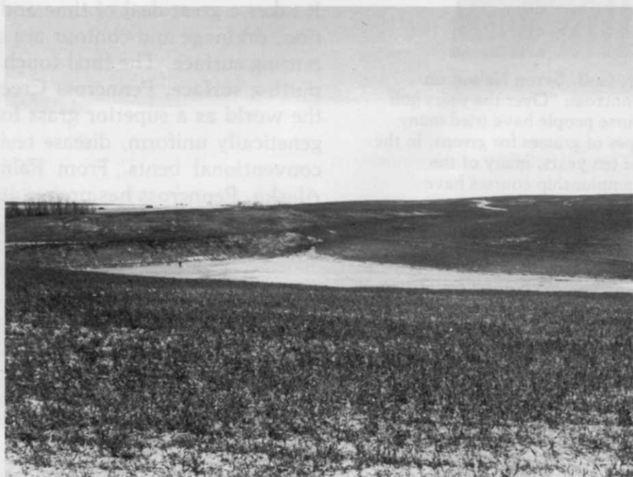
Workers for the Ohio Mining and Reclamation Association prepare to mulch newly seeded area nearby (top). A silt basin (below) is a vital part of mine reclamation and is usually the first step of the reclamation process. Reclaimed soils can absorb limited quantities of rainfall. Therefore, increased runoff must be handled through special ditches and silt basins.
