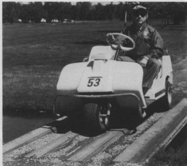
Golf cart tires fit the grooves created by four sheets of piling. Gravel placed in grooves allows golfers to avoid the grinding of cleats on the metal sheeting.
