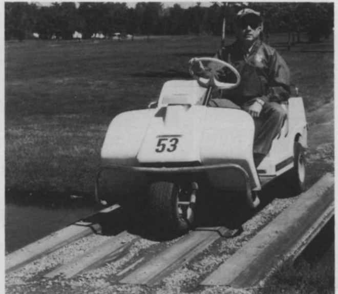
Golf cart tires fit the grooves created by four sheets of piling. Gravel placed in grooves allows golfers to avoid the grinding of cleats on the metal sheeting.
